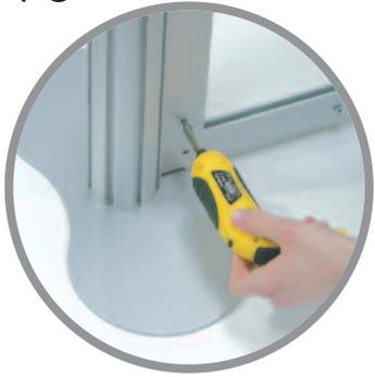
Connect side vertical rails to the bottom horizontal rail. The side vertical rails have one run of tape on them. Strip should be nearest the post when viewed from the front.
